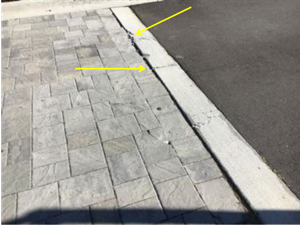
Photo 78- pavers and concrete at entry gate
