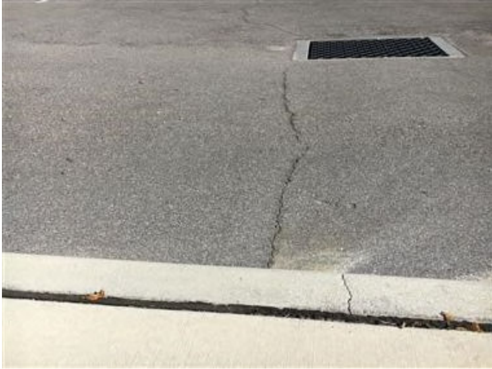
Photo 60- asphalt parking and curb
