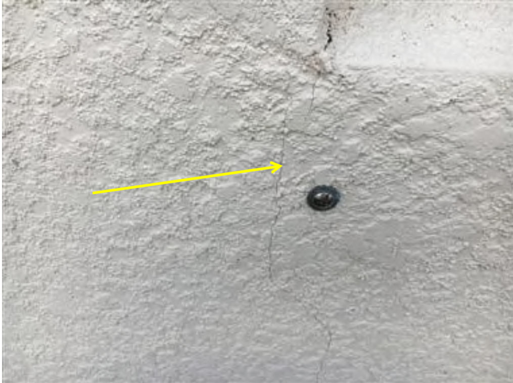
Photo 95- wall cracks
