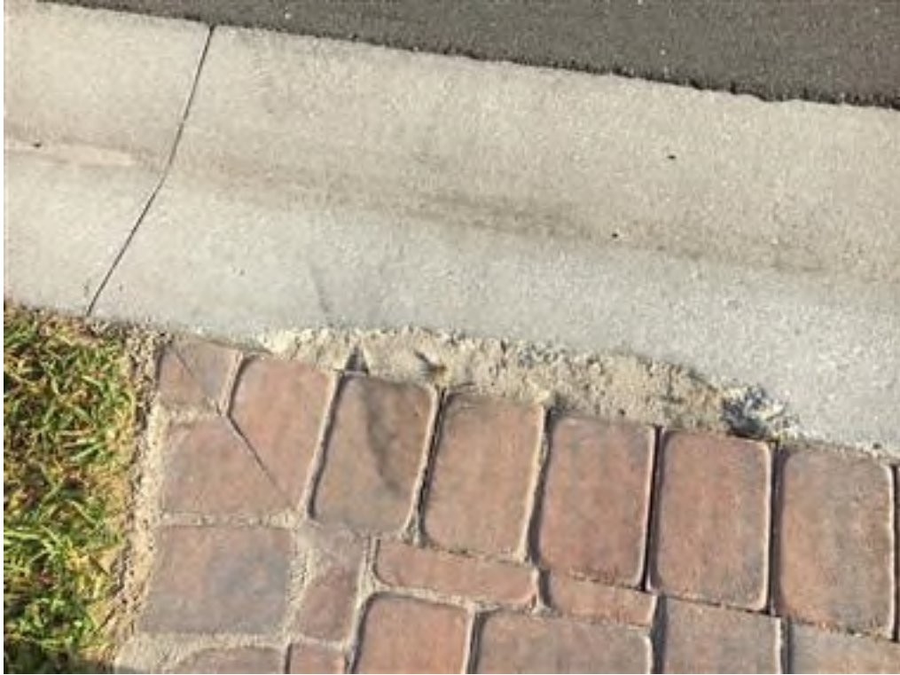
Photo 86- concrete curb, typical
