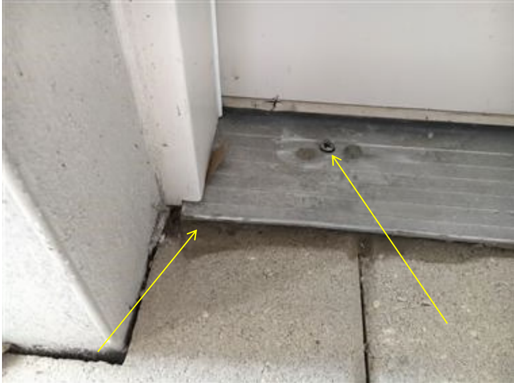
Photo 31- pool area restroom
