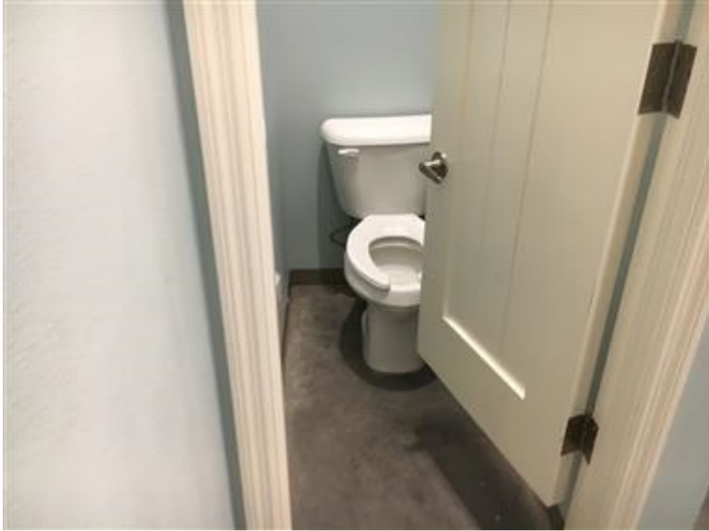
Photo 30- pool area restroom
