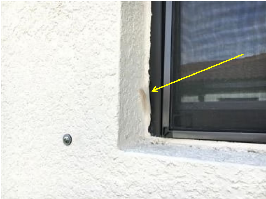
Photo 105- window sealant typical 9835 Haze Drive
