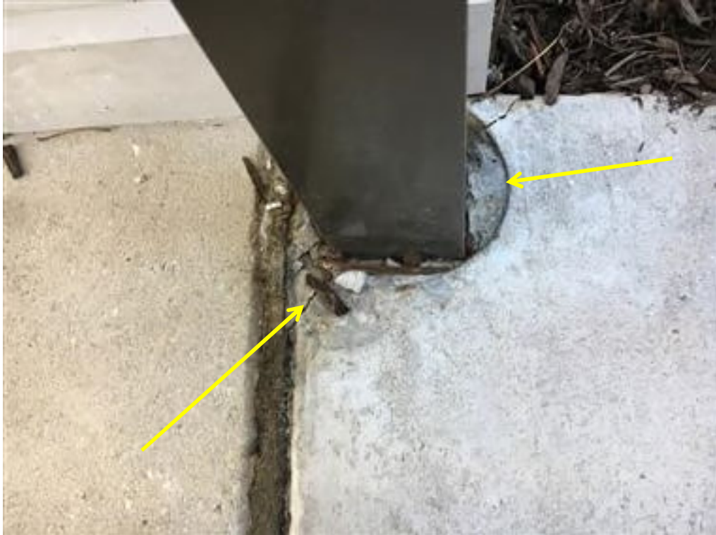
Photo 39- gate post pocket
