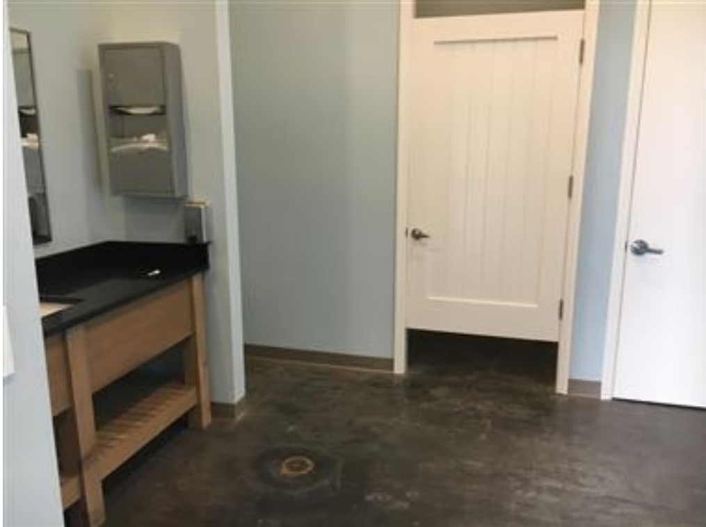
Photo 25- pool area restroom
