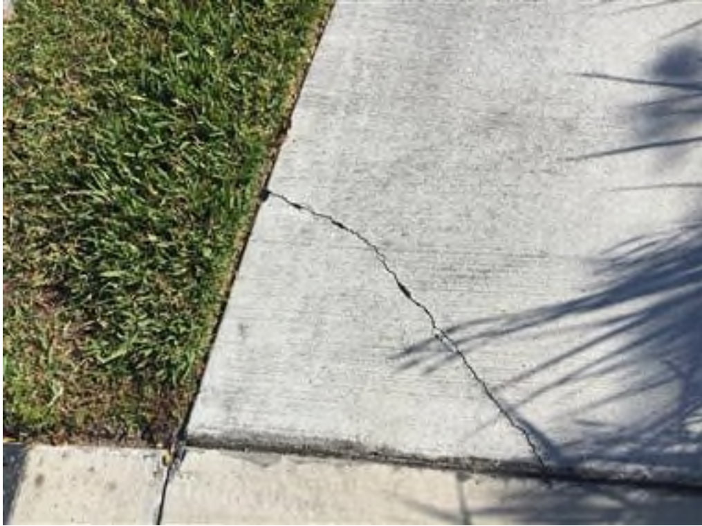
Photo 62- sidewalk near clubhouse
