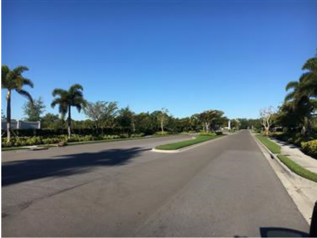
Photo 132- asphalt paving at entry
