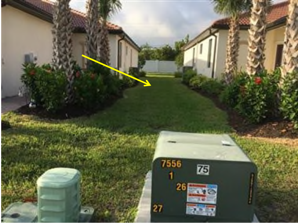
Photo 88- swale area 9851-9847 Haze Drive
