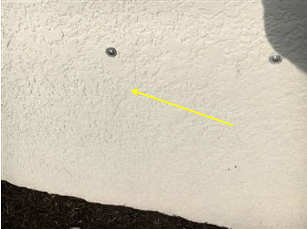
Photo 97- wall cracks
