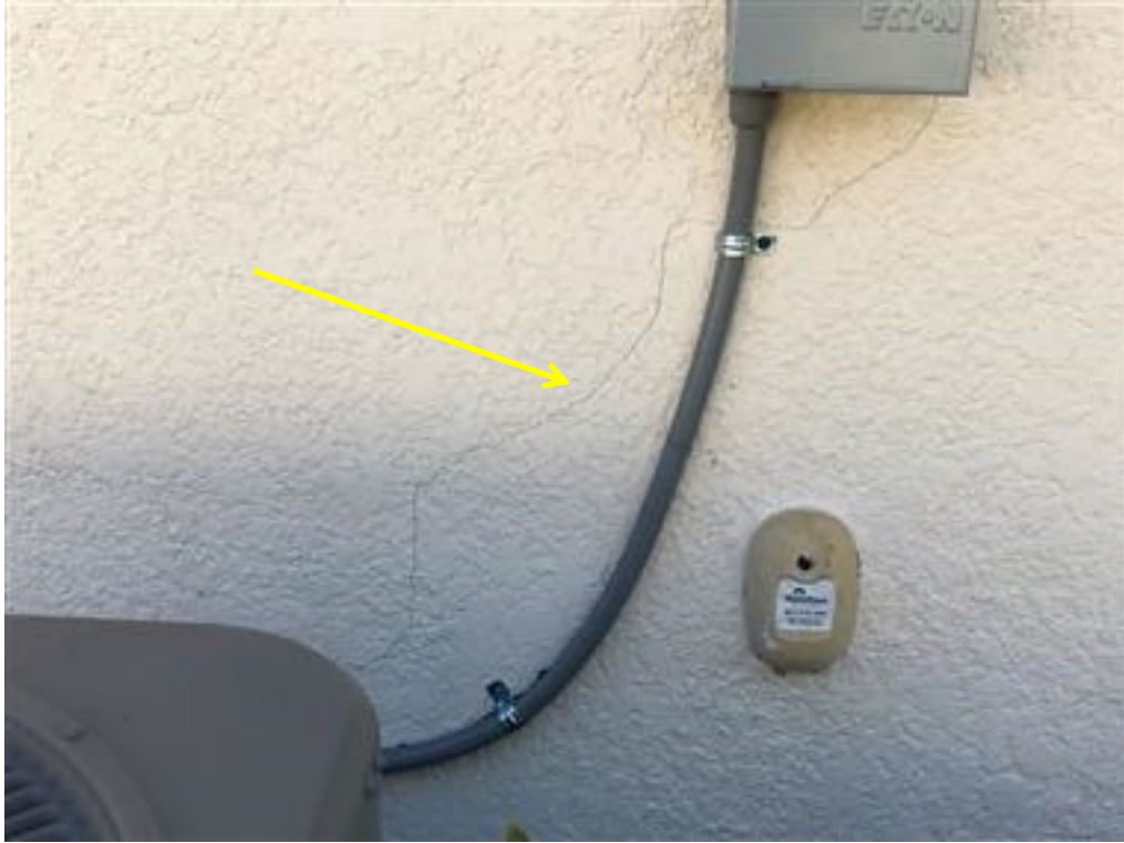
Photo 96- wall cracks
