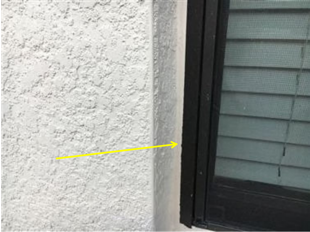
Photo 94- sealant at window
