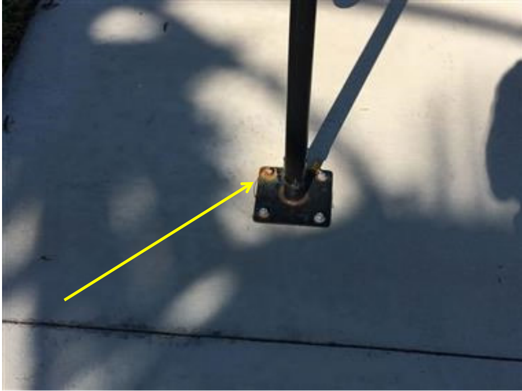
Photo 64- rusted fasteners
