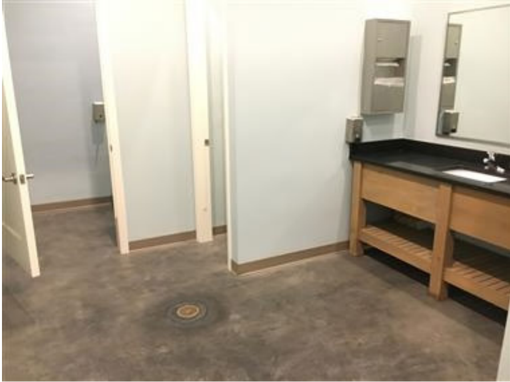
Photo 28- pool area restroom
