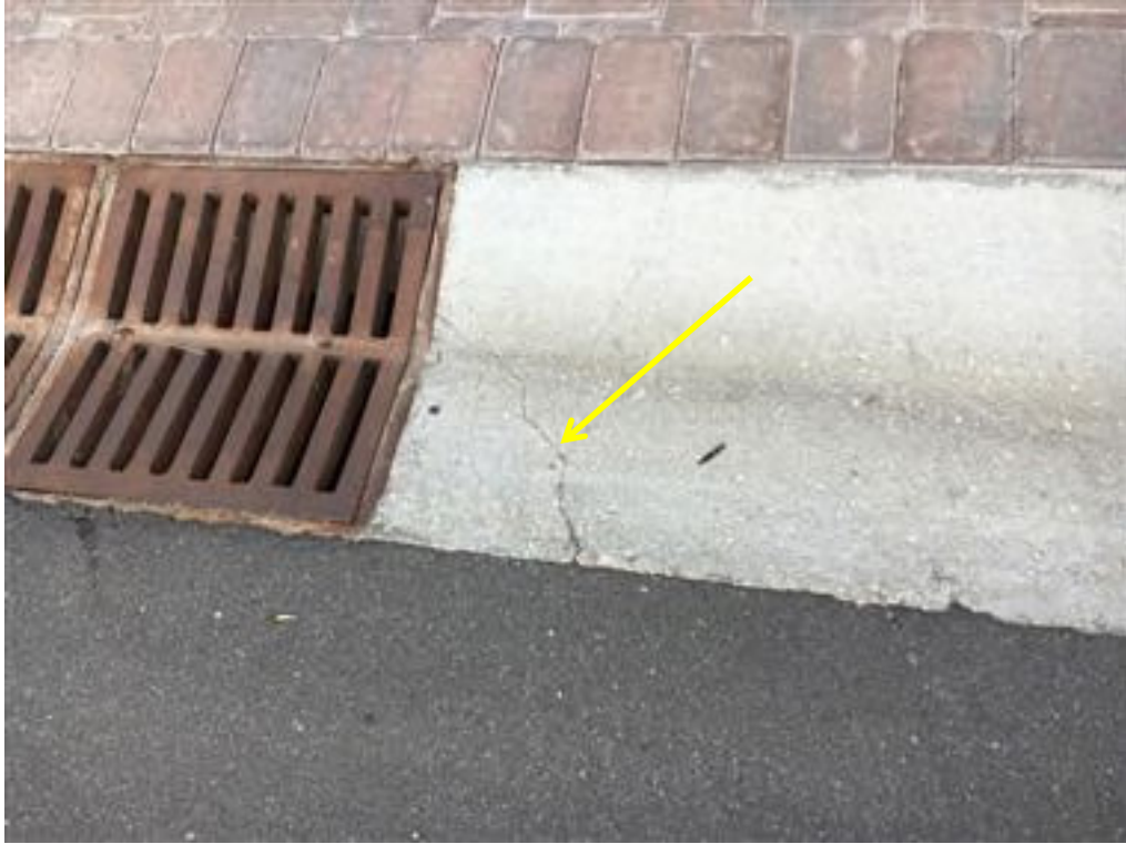
Photo 108- concrete curb, typical
