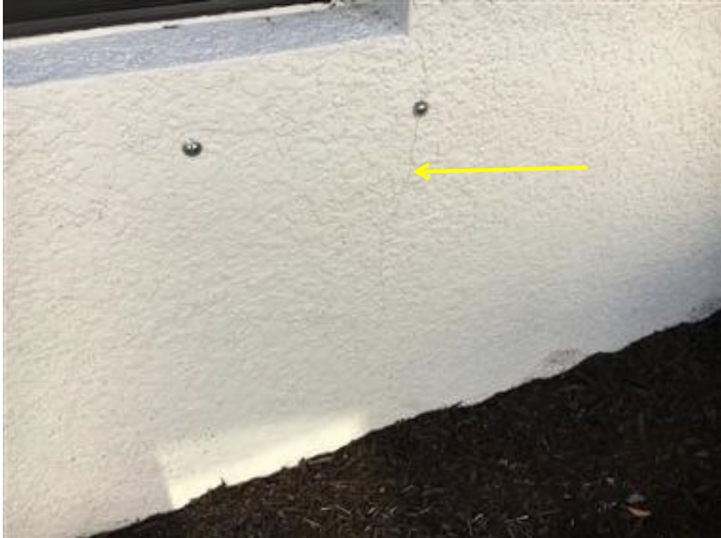
Photo 99- wall cracks
