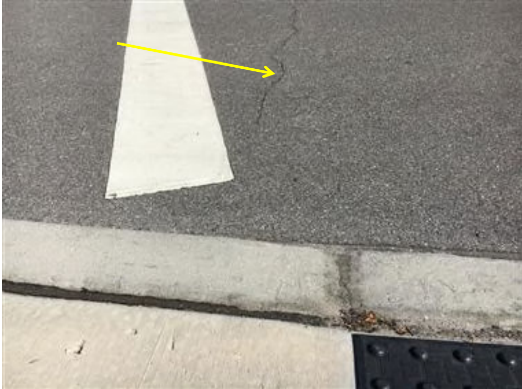
Photo 57- asphalt parking and curb
