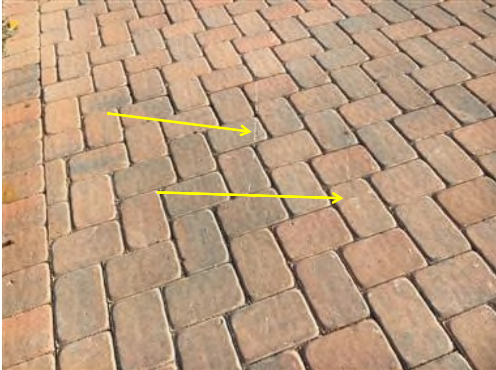
Photo 85-pavers with cuts 9851Haze
