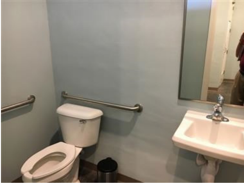
Photo 26- pool area restroom
