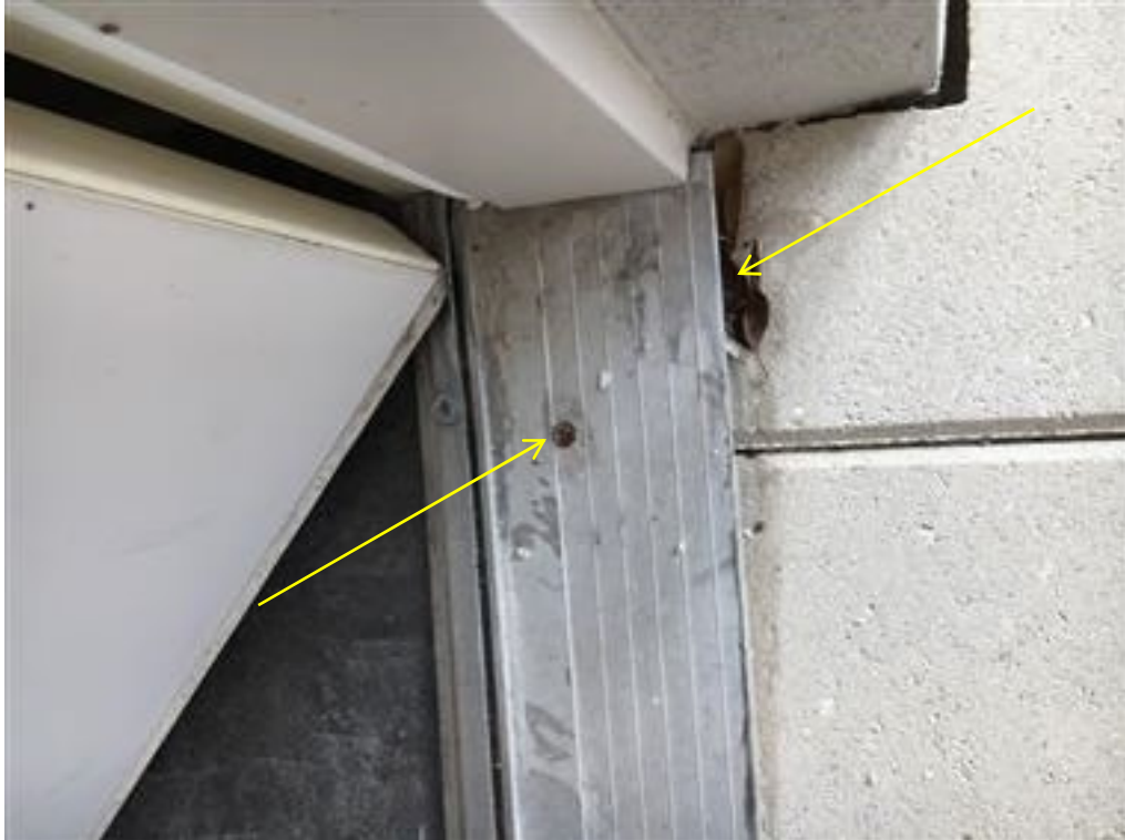
Photo 27- pool area restroom
